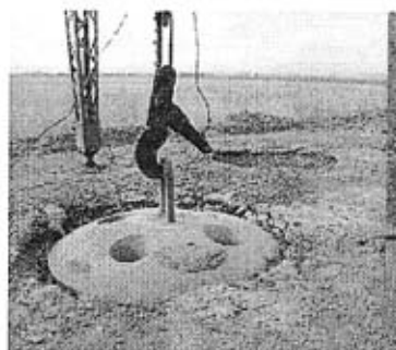
图 1.2-3 夯锤及脱钩装置 Fig1.2-3 Rammer and separating device
